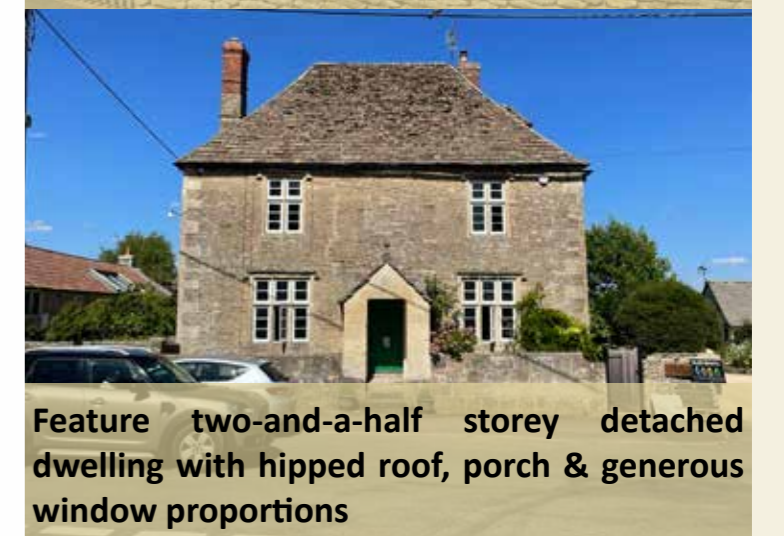
Limestone cottage with stone slate roof, brick chimney & simple stone detailing, characteristic of Kington
