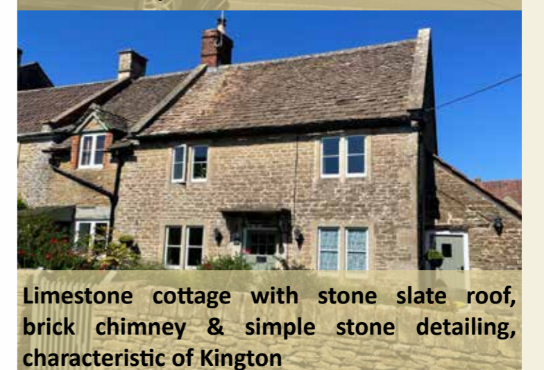
Traditional stone cottages with coursed rubble walls, steep stone slate roofs & prominent brick chimneys
